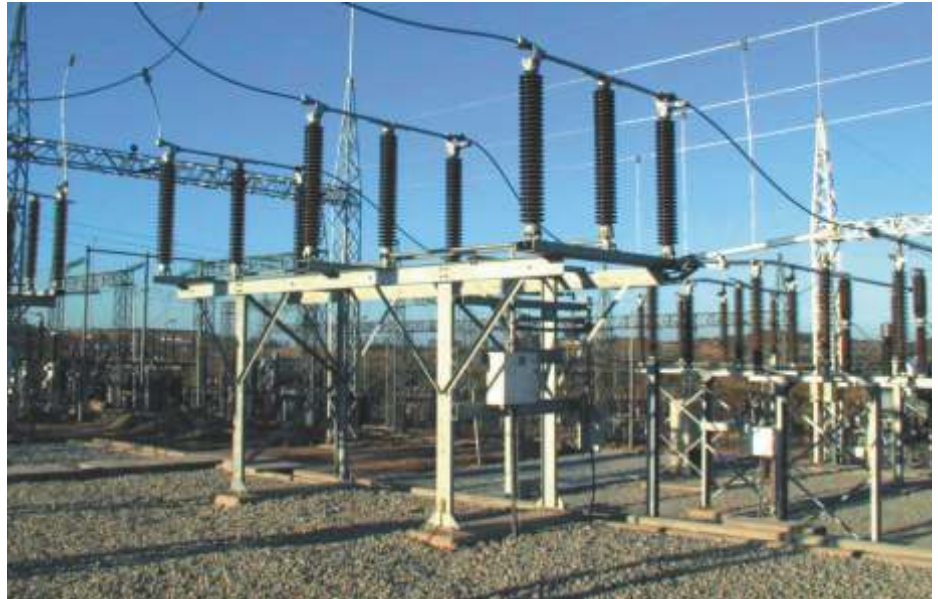
A 132 kV/1 600 A, 650 kV double side break motorised disconnecter.
