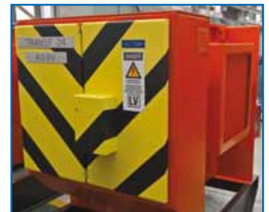
Figure 5, LV panel enclosure IEC 62271-202
