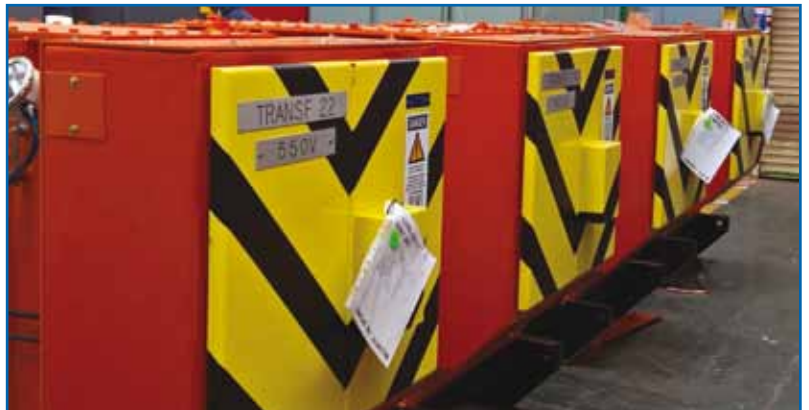
Figure 3, typical skid base type minisub
