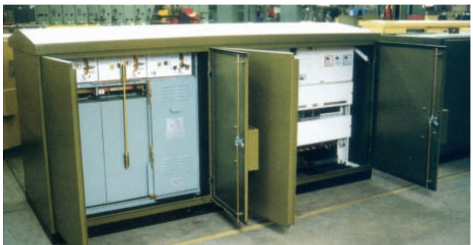
*Type B miniature substation with all compartment doors open.
