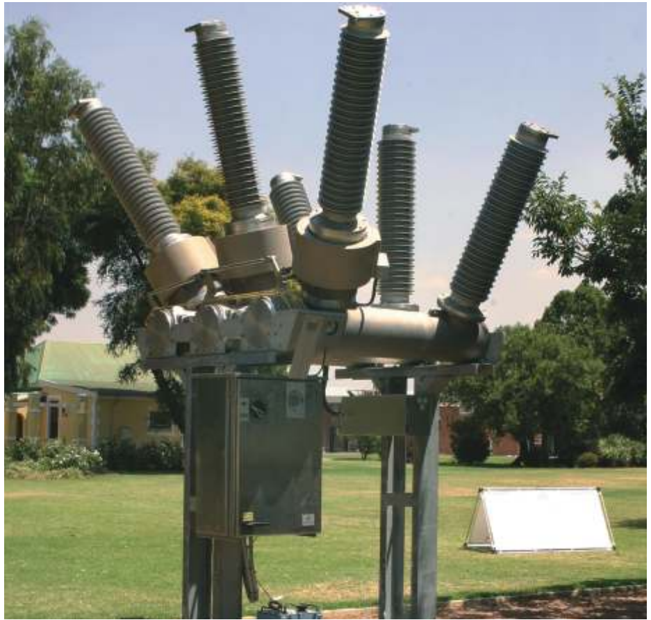
HYpact switchgear.
